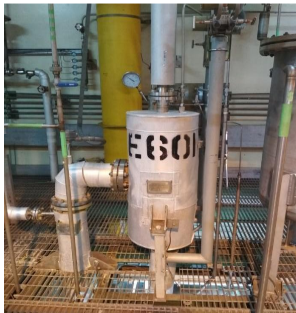
Gambar 1. Vertical Tube Evaporator
