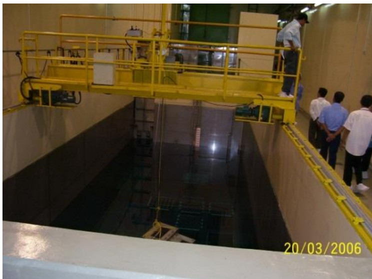
Figure 1. The pool of ISSF in Serpong Area
