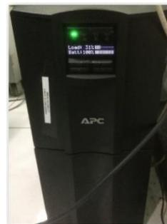
**Gambar 2. Kapasitas UPS 5kVA SIK reaktor**
