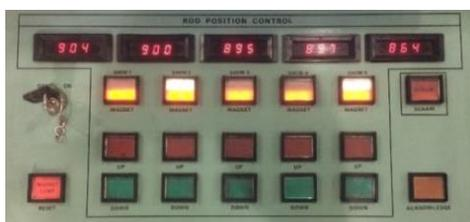
**Gambar 5. Panel kontrol batang kendali reaktor**
