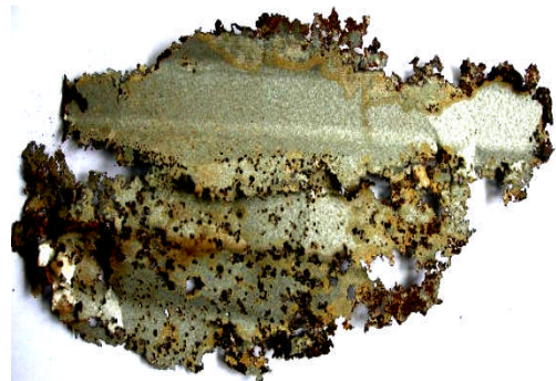
Figure 1. The corroded Al-Zn heat reflector.
