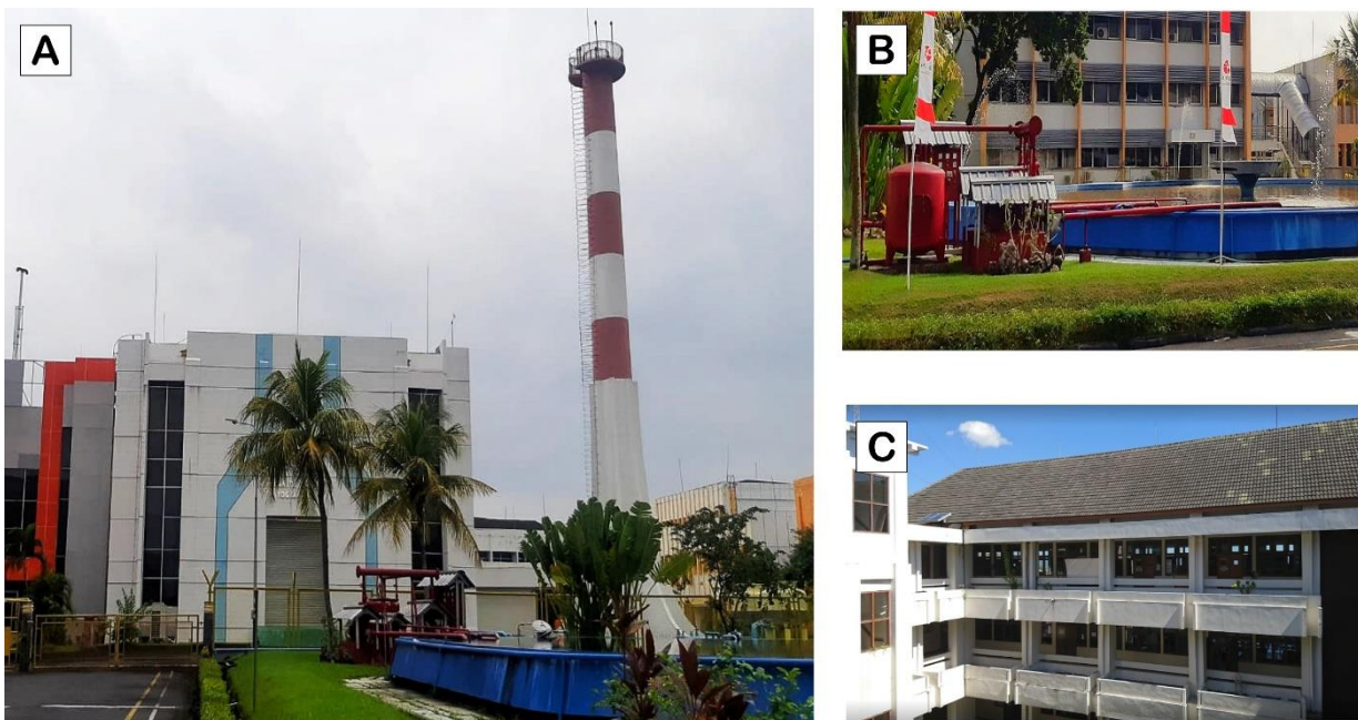
Figure 4. Infrastructure buildings in the Yogyakarta Nuclear Area.
