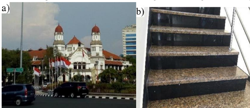
Figure 3. a) The granites used in building the Lawang Sewu actually originated from Europe.[6]; b) Cracks in granite can be overcome by polishing techniques so that they can be used as small expensive ornaments [26]
