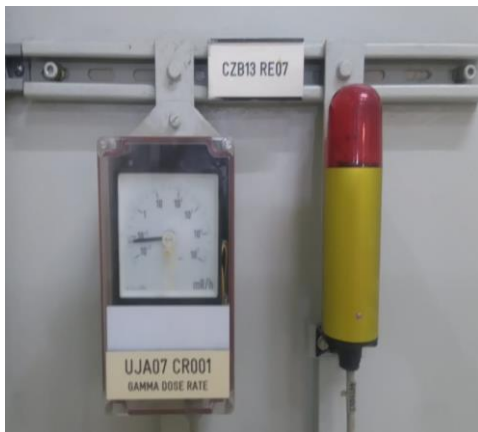
Gambar 3. sistem Alarm Unit Emergency
